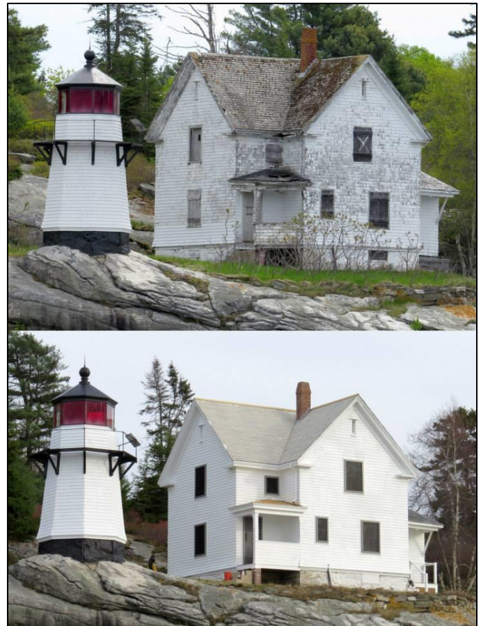
Perkins Island lighthouse and keeper’s house before and after restoration work. Photo – American Lighthouse Foundation
