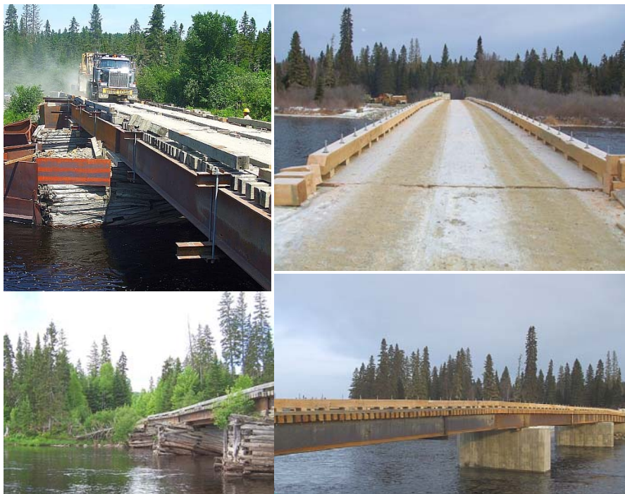
Before and After – Reconstruction of the Henderson Brook Bridge, Allagash Waterway
