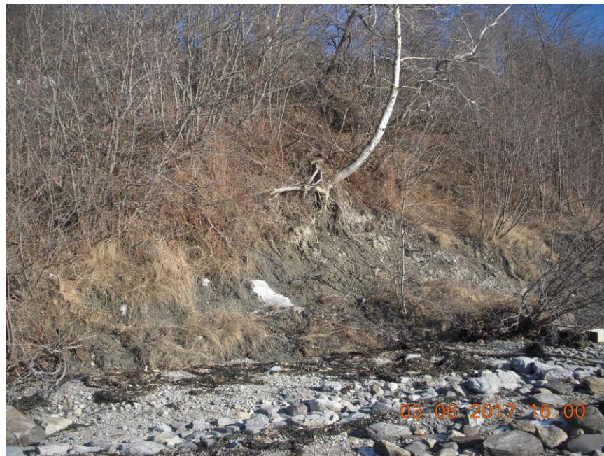
Figure 13. A section of eroding bluff at Mitchell Field shows exposed glacial till and slope creep in a birch tree trunk. Toe erosion here could be mitigated with revegetation, tree wads, and cobble beach nourishment. Photo by S. M. Dickson.
