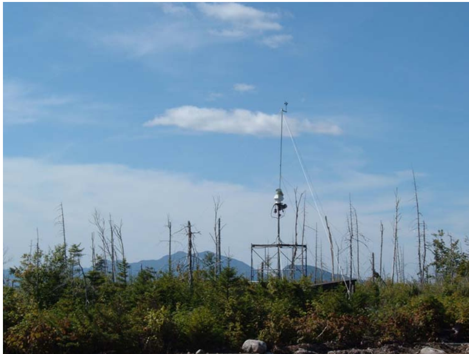
Figure 2-6. Radar situated in Highland Project area.
