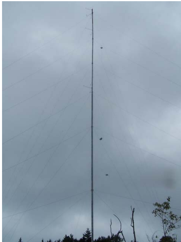
Figure 3-2. Typical view of acoustic bat detectors deployed from met tower guy wires.
