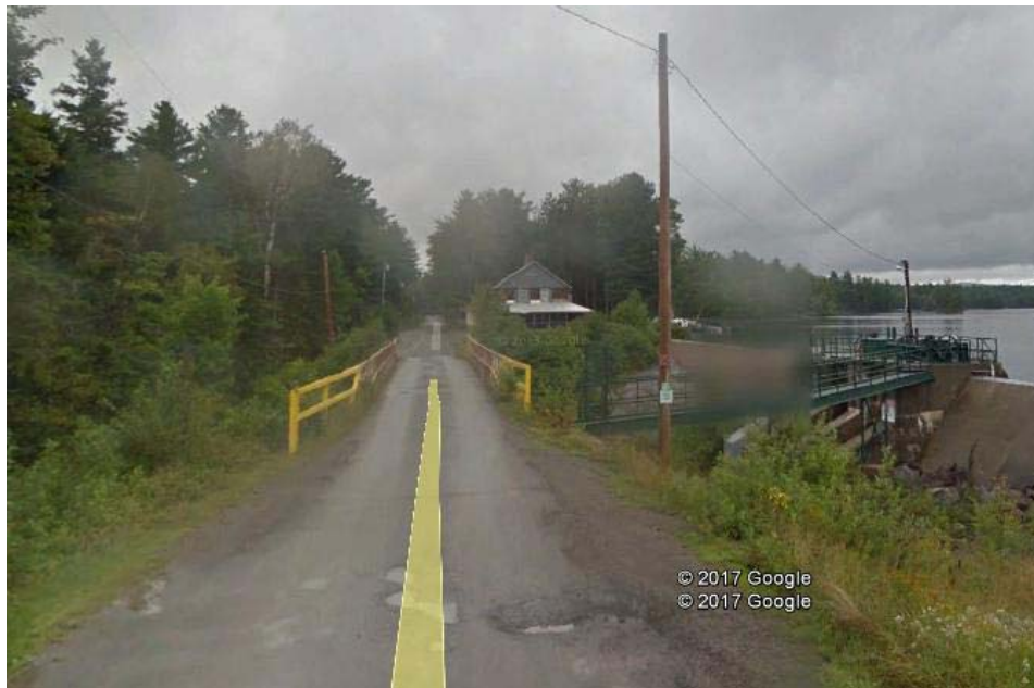
Eastern Access: One-Lane Bridge near East Moxie
