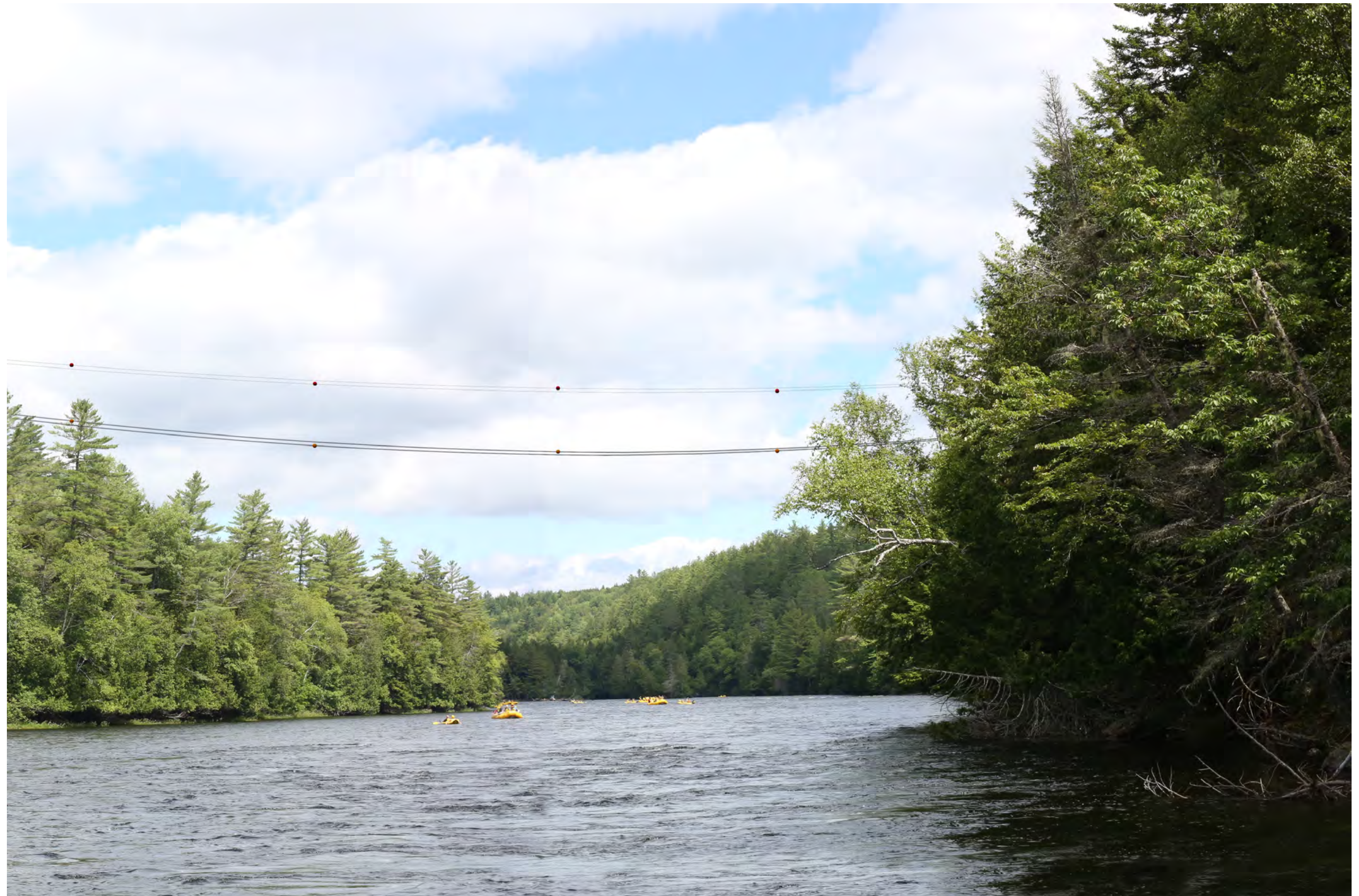
Proposed Conditions: Normal view looking northeast from near the picnic area on the Kennebec River 1,400'+/- south of the proposed HVDC transmission line crossing. The lowest point of the conductors would be approximately 200' above the water level. Approximately eighteen marker balls will be placed on the shield wires and conductors above the Kennebec Gorge.
